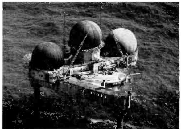
The Dresser-Ideco radar antenna structure in the center of the deck of this Texas tower is another example of the variety of towers designed and fabricated by Dresser-Ideco's large, diversified Tower Division. This installation is off the north Atlantic coast, east of Cape Cod.
